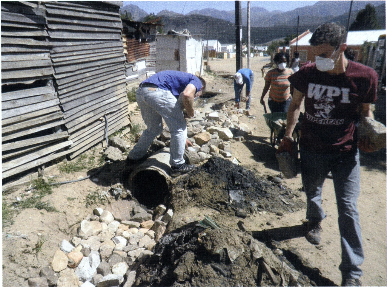
FIGURE 4 Shaping Place Through Informal Stormwater Channels
