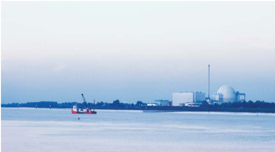
Fig. 1: Unterweser nuclear power station
