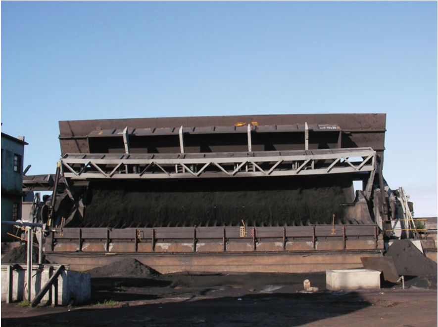
Tippler operation in Mozambique Port
