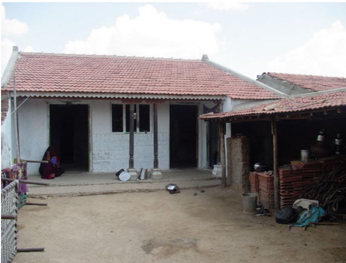
Figs. 7.1 and 7.2 Owner-built houses in Gujarat (Source: Duyne Barenstein)
