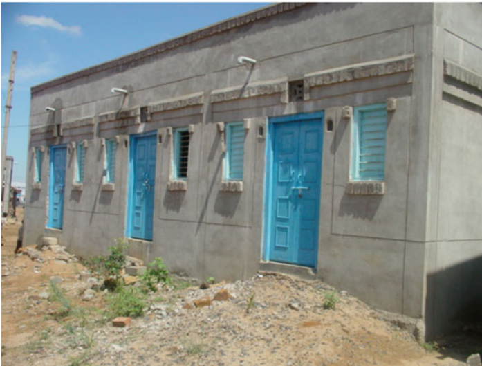
Figs. 7.3 and 7.4 Contractor-built houses in relocated sites in Jamnagar District, Gujarat (Source: Duyne Barenstein)
