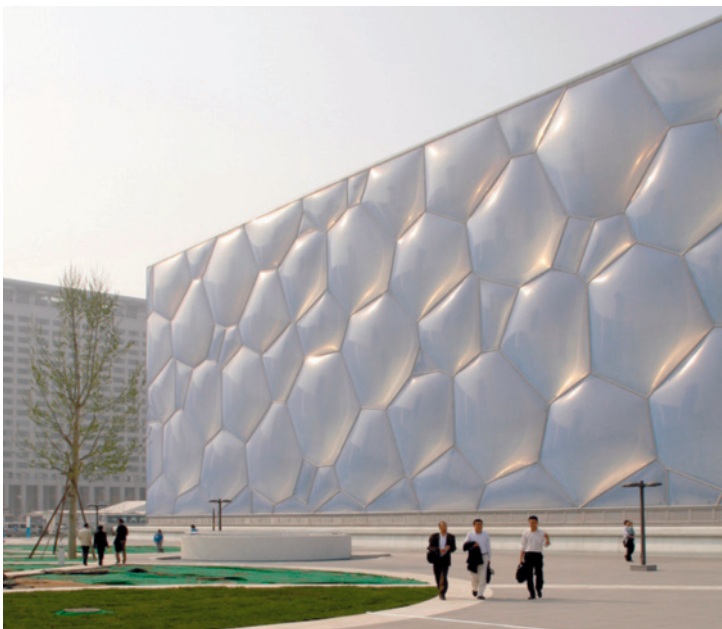
Fig. 4. The outer skin of the building is made of ETFE membrane cushions
