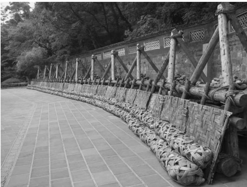
Fig. 1.4 Model of a water control structure used in the Dujiangyan irrigation system, now part of a United Nations World Heritage Site. Photo by authors. (A color version of this figure appears between pages 72 and 73.)
