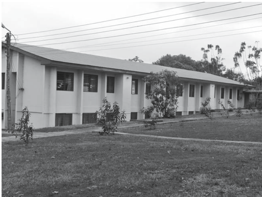
Figure 1.4 Forest Biology building at the Forestry Research Institute of Ghana at Fumesua, near Kumasi. Both the Entomology and Pathology Sections are located in this building
