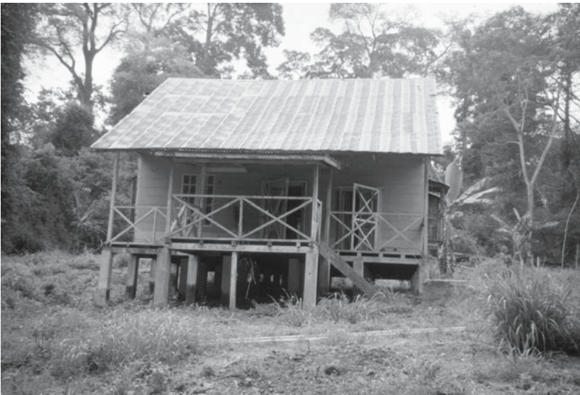
Figure 1.2 Old wooden guesthouse at Bobiri Forest Reserve and Butterfly Sanctuary. Structure was constructed c.1940 with termite- and wood decay-resistant tropical trees
