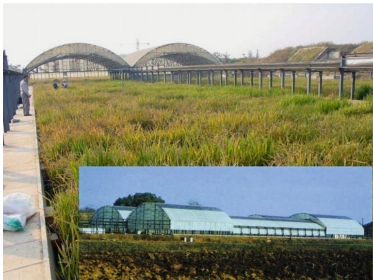
Fig. 4.4 A large motorized moveable rainout shelter at the National Key Laboratory of Crop Genetic Improvement, Huazhong Agricultural University, Wuhan, China. Rice experimental materials grow in the protected area while the shelter is parked on the two edges of the protected area. Inset: The installation set at full cover
