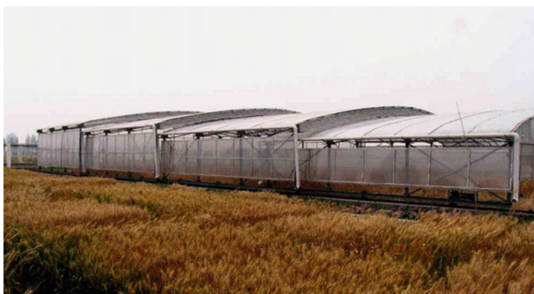
Fig. 4.5 Multi-cover installation combined of 4 roof sections set over the protected plot. Each section travels on its own tracks and sections are parked towards the far end one under the other when they are off the protected plot. Notice the water drains on each section (The Luoyang Station of the Luoyang Academy of Science, Henan China)
