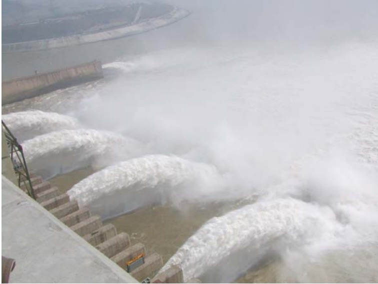
(A) Bottom outlet operation on 20 October 2004— Q = 1700\text{m}^3/\text{s} per jet, V = 35\text{ m/s} (Shutter speed 1/1,000\text{ s} ).
