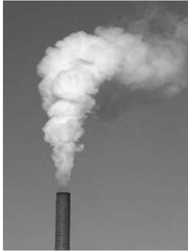
Figure 1.2. A smokestack plume. Note the turbulent billowing inside the plume, which is the cause of its gradual dispersion in the ambient atmosphere. (Photo by the first author).
