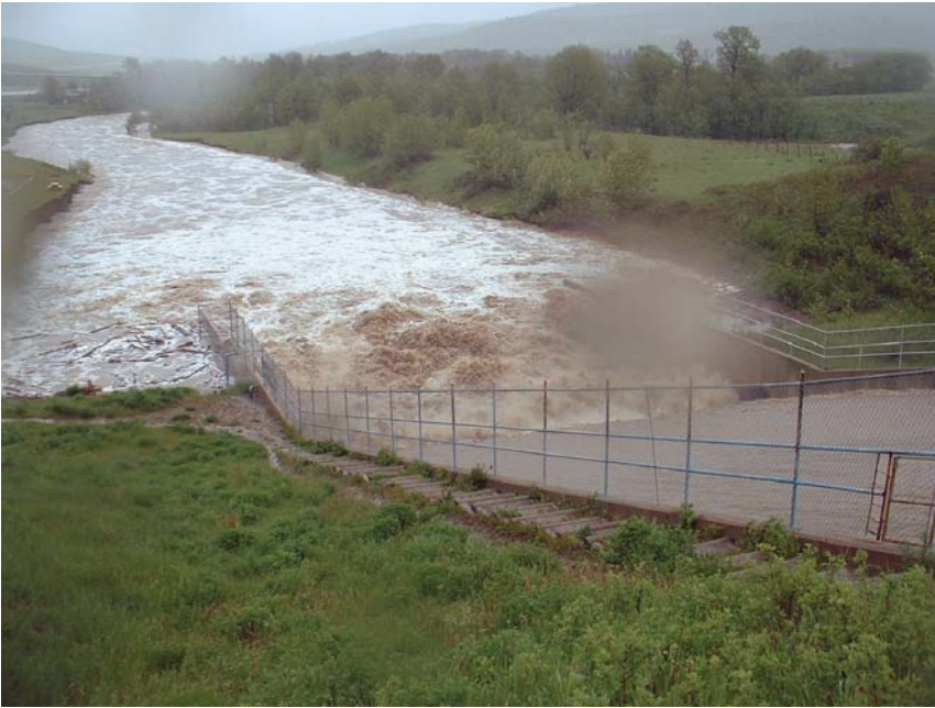
Figure 7.2. Air bubble entrainment in a hydraulic jump at the downstream end of a spillway chute—Chain Lakes dam spillway, Southern Alberta, Canada, June 2005 (Courtesy of John Rémi)—Looking downstream, with a discharge of about 300 \text{ m}^3/\text{s} —Note the “brownish” dark colour of the flow caused by the suspended load and the “white” waters downstream of the hydraulic jump highlighting the air bubble detrainment.
