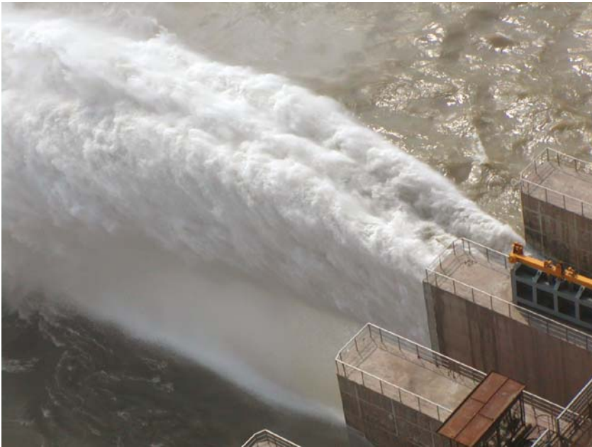
(B) High-velocity water jet at Three Gorgas dam—9 m by 7 m jet, V_1 = 35 m/s, high-shutter speed (1/1,000 s)
