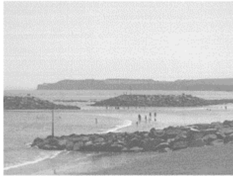
Plate 8.3: Sidmouth, England. Beach erosion protection.
