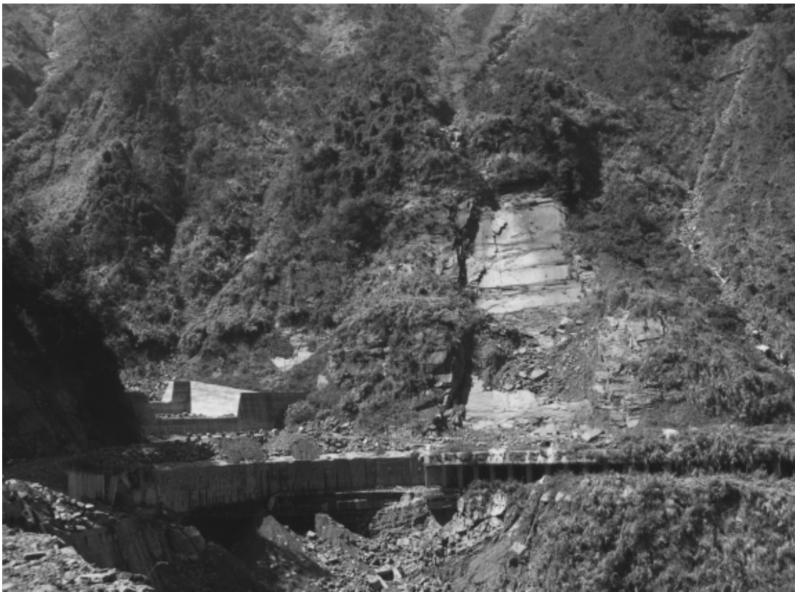
Plate 8.1 A landslide on a road in central Taiwan caused by erosion exposing a plane of weakness in the rock mass. Note that the road has been protected using an avalanche shed, but the whole road has subsequently been destroyed by a debris flow induced by a typhoon.
