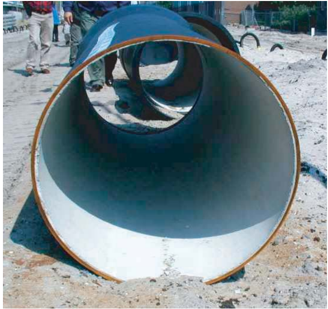
Figure 4.34. Cement lined DI pipe with PE coating.
