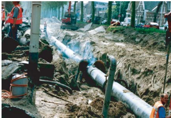
Figure 5.1. Laying of steel pipe.
