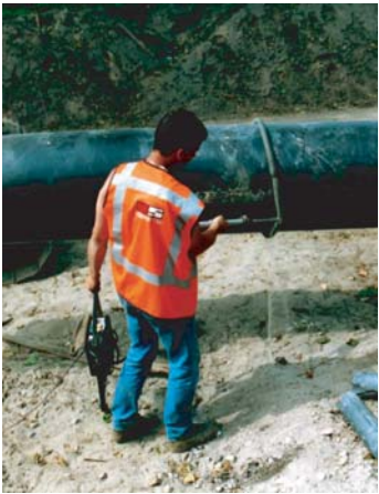
Figure 5.12. Testing of external coating.
