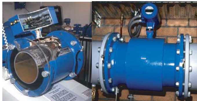
Figure 4.59. Magnetic meters (Manufacturer: Krohne).
