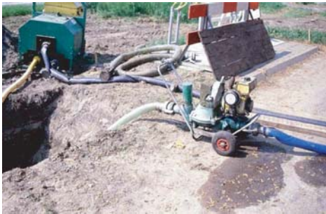
Figure 5.7. Trench dewatering by pumping.
