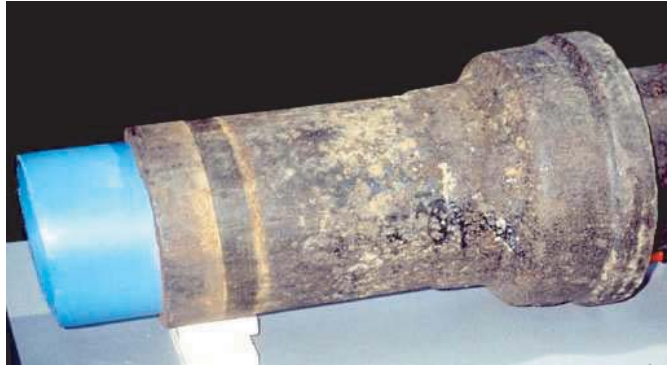
Figure 6.40. Structural relining of an old CI pipe.
