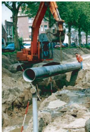
Figure 5.13. Pipe positioning in a trench.
