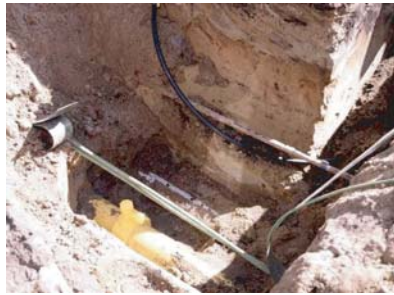
Figure 5.4. Manually excavated trench.
