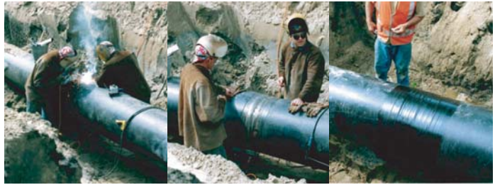
Figure 4.44. Welding of steel pipes.
