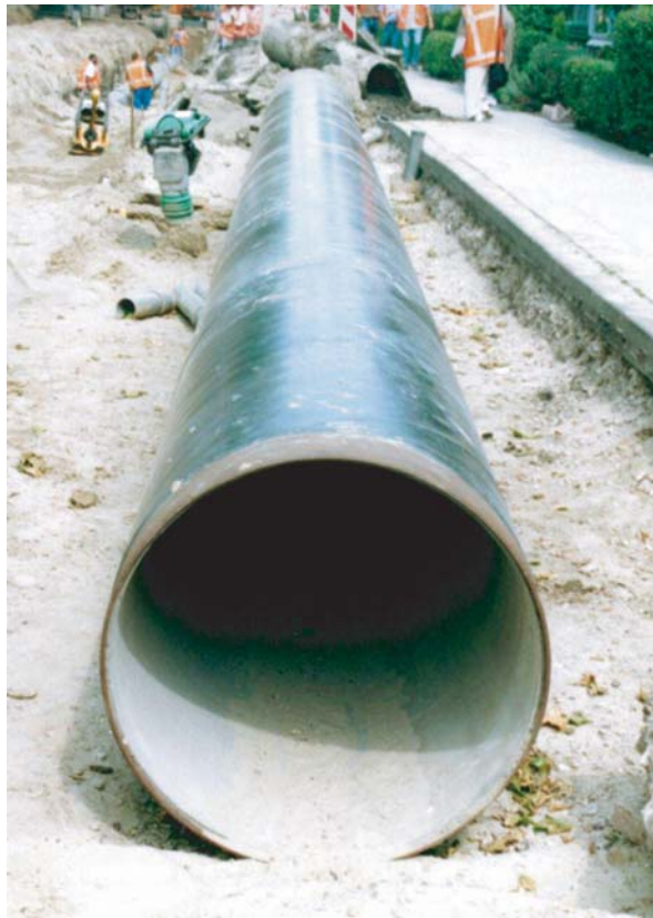
Figure 4.36. Cement lined steel pipe with PE coating.
