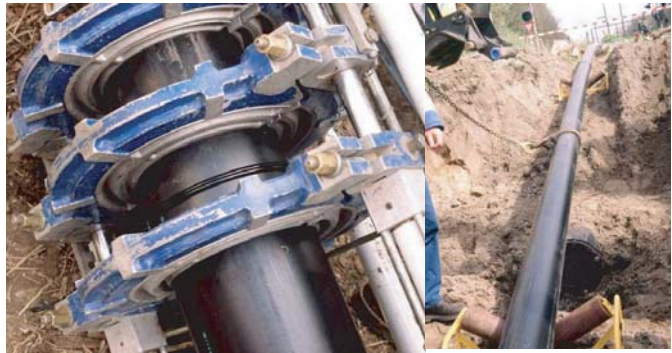
Figure 4.45. Welding and laying of PE pipes.
