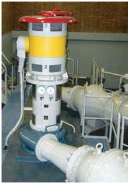
Figure 1.15. Vertical centrifugal pump.
