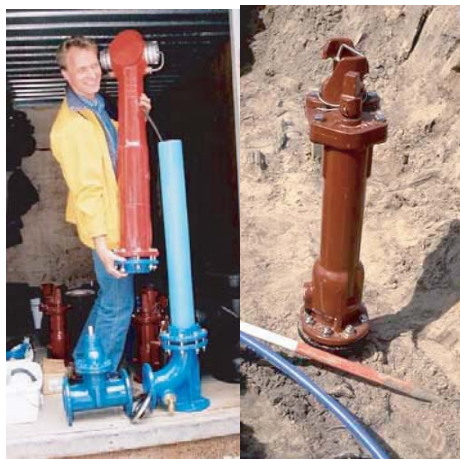
Figure 4.66. Ground level- and underground fire hydrants.
