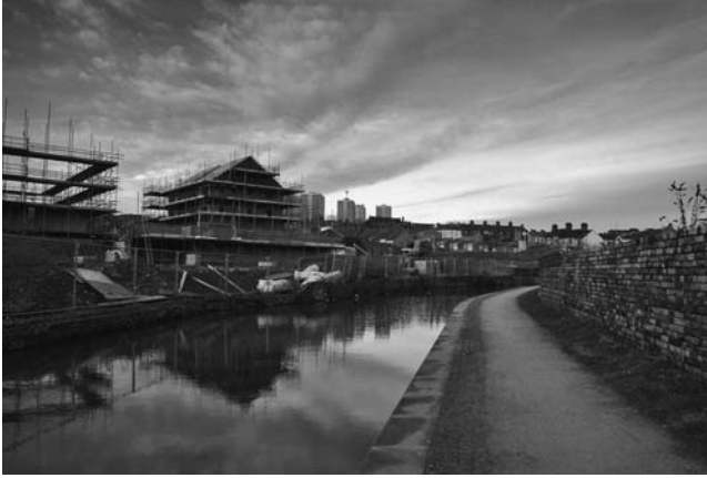
Figure 12 New housing along the Caldon canal where potbanks previously stood.
