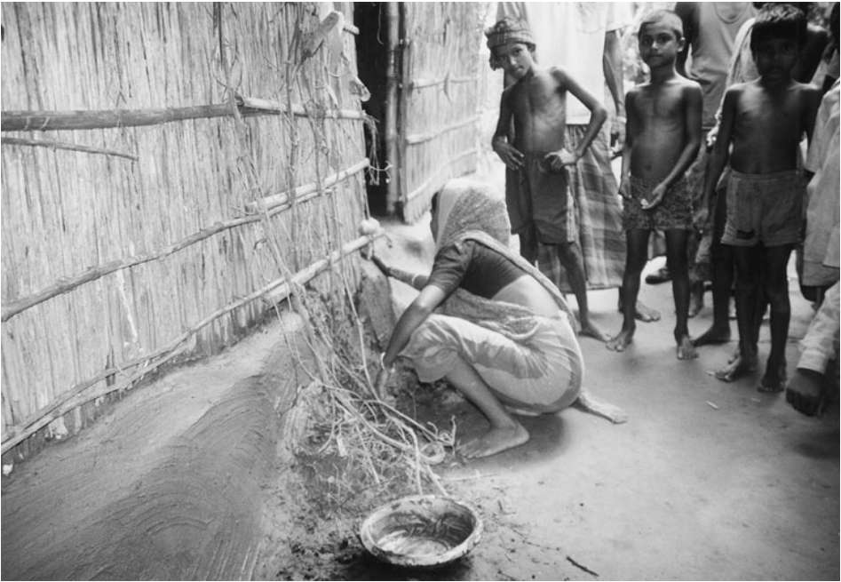
Plate 5.5 Bangladesh: a woman applying a new layer of mud to strengthen the foundation of her house during the monsoon season, when flooding is common. Her husband is a handloom weaver as the family has no land, so the wife is responsible for all outdoor work as well as housework and childcare.
