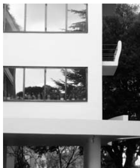
2.10 Highpoint, Highgate; detail of entrance canopy: Berthold Lubetkin and Tecton, published in Architectural Review , January 1936.
