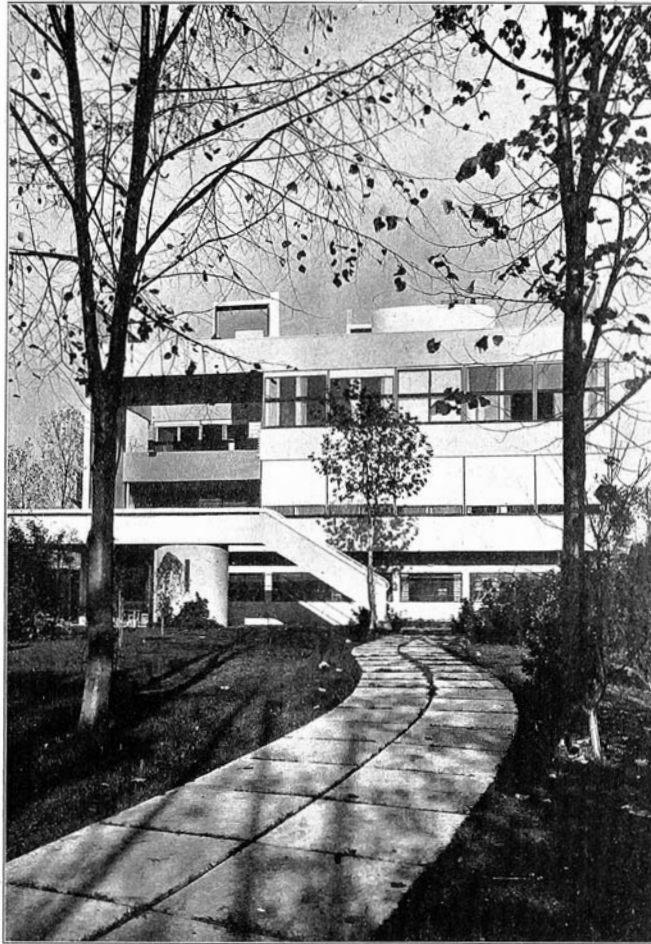
"LES TERRASSES" GARCHES: THE GARDEN FRONT, WITH ITS TERRACES AND OUTSIDE STAIRCASE. LE CORBUSIER & JEANNERET, Architects.
