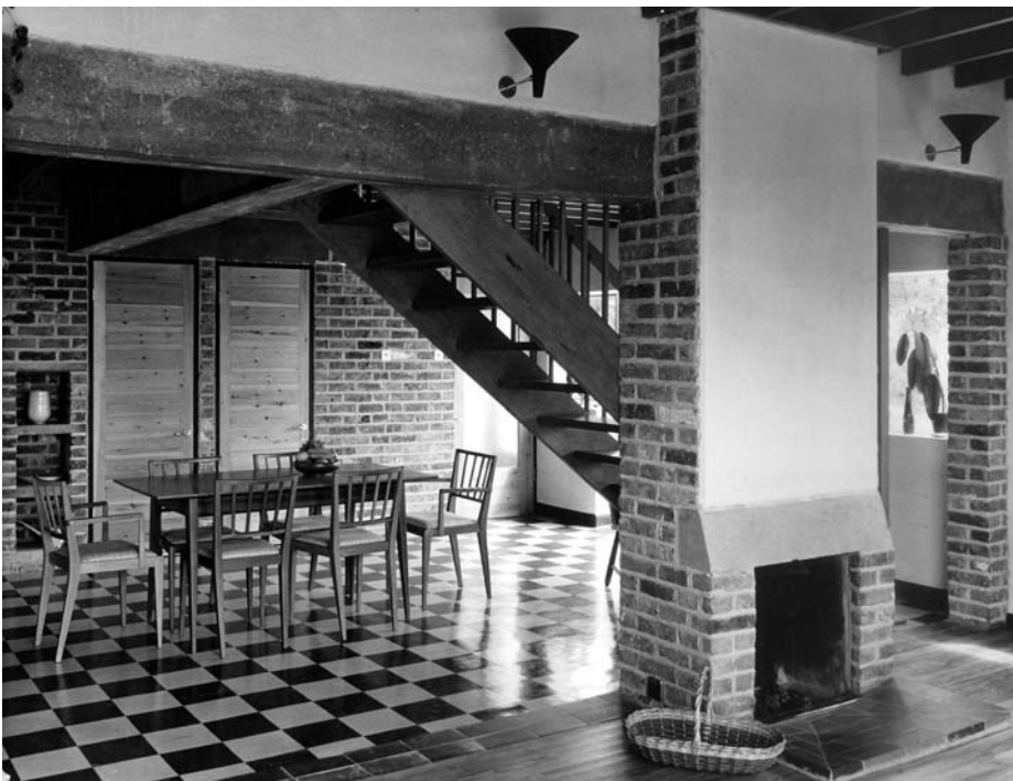
4.4 Interior of Sugden House, Watford 1956; Alison and Peter Smithson, with unplastered stock brick and untreated timber.
