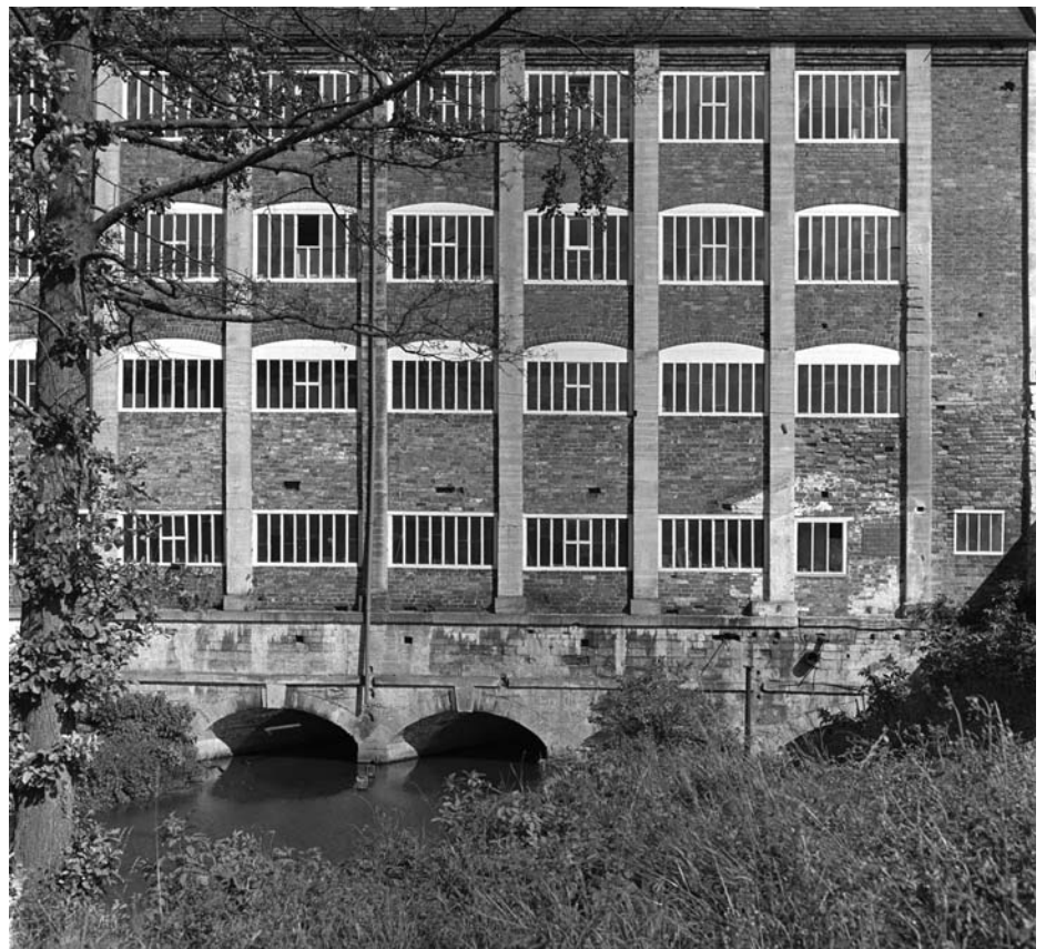
4.8 Eric de Maré: photograph of Stanley textile mill 1813, Stroud Valley, Gloucestershire used in The Functional Tradition in Early Industrial Buildings, 1958.
