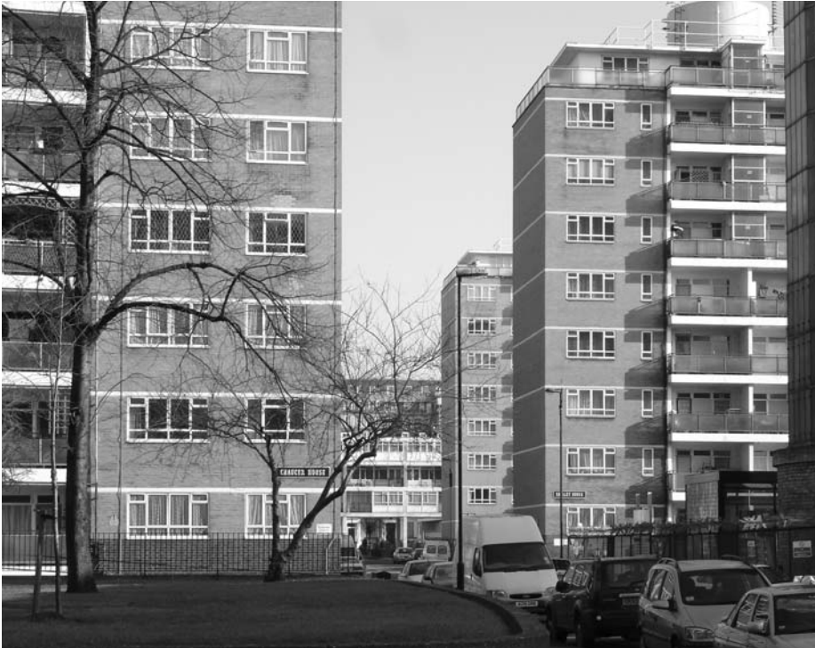
3.8 Churchill Gardens, Pimlico designed by Powell and Moya 1946 and consistent with the Abercrombie Plan's reconstruction principles, showing blocks in the earliest section built 1950
